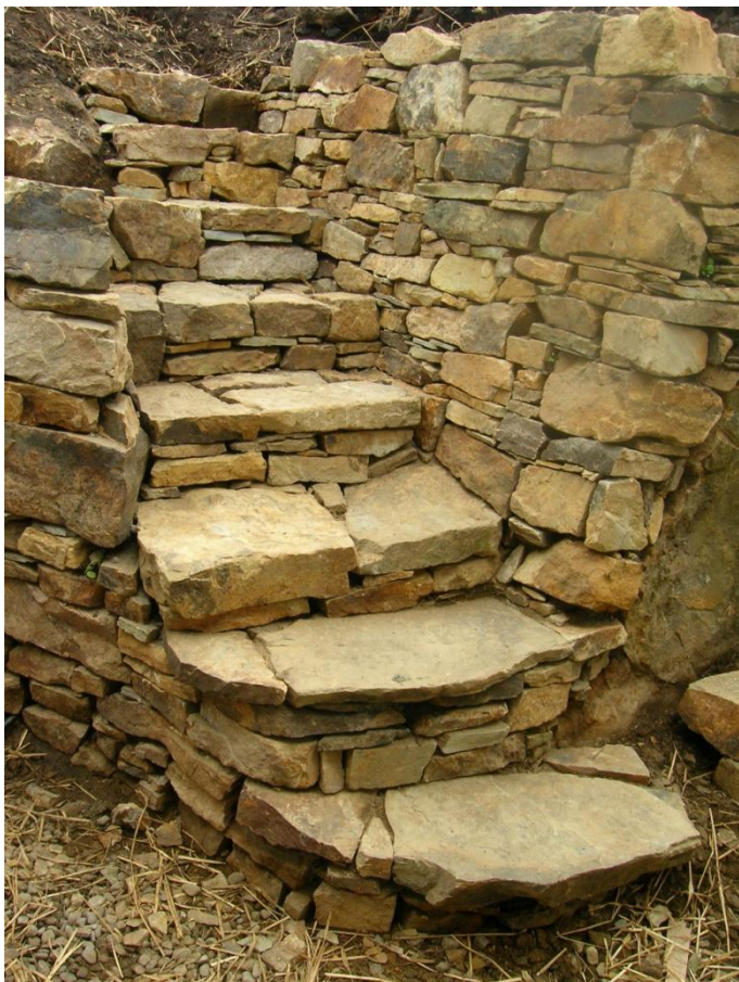
Stone steps being built
